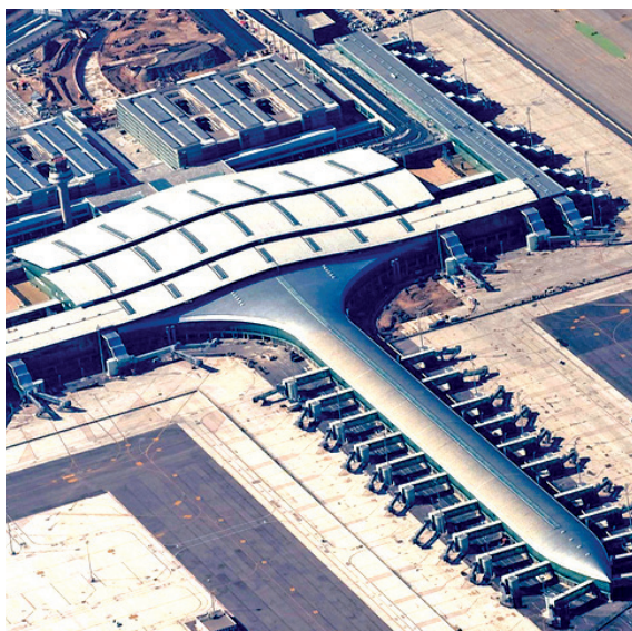
T1 Barcelona Airport – Arq. Ricardo Bofill
